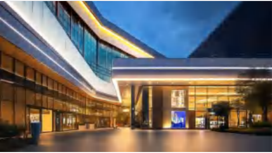
General Lighting for Commercial and Office Spaces
